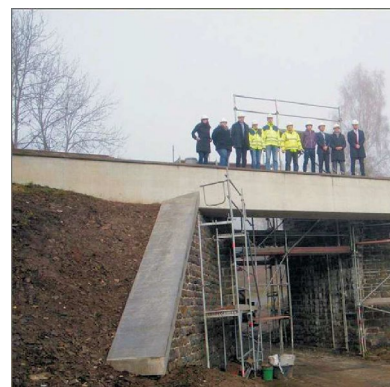
Figure 23: A public bridge built out of futurcement/futurconcrete.
